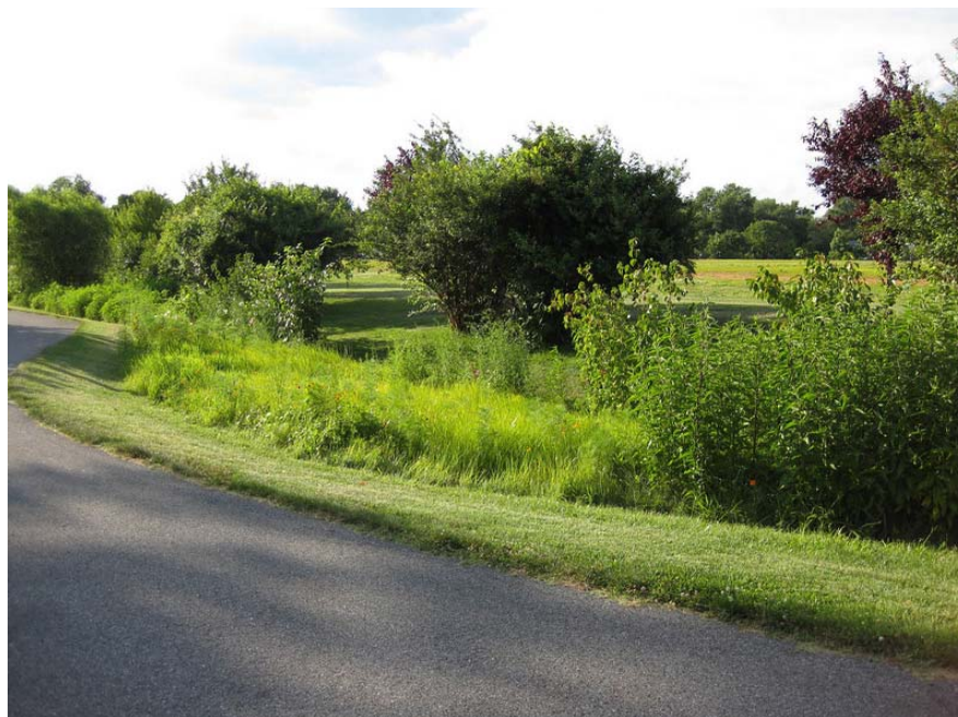
Figure 5.2. Water Quality Swale w/ tall meadow grasses & herbaceous plants along trail receiving runoff from parking area (source: National Transportation Enhancements Clearinghouse / www.enhancements.org )
