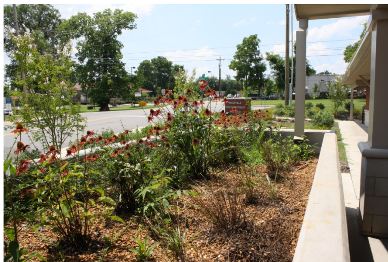
Figure 2.1. Stormwater Planters
