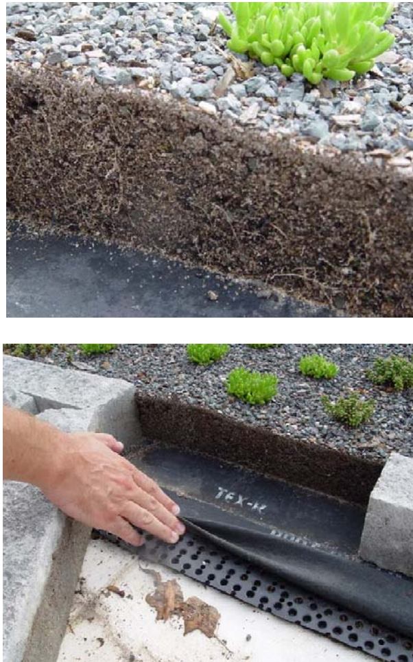
Figure 12.1. Photos of Vegetated Roof Cross-Sections (source: B. Hunt, NCSU)
