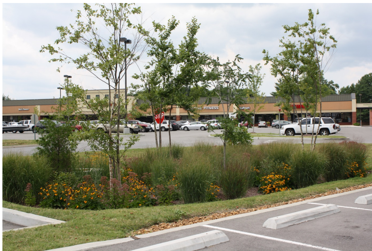
Figure 1.1. A Typical Bioretention Basin treating a parking lot.
