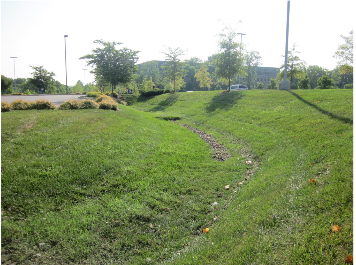
Figure 8.5: Typical Grass Channel
