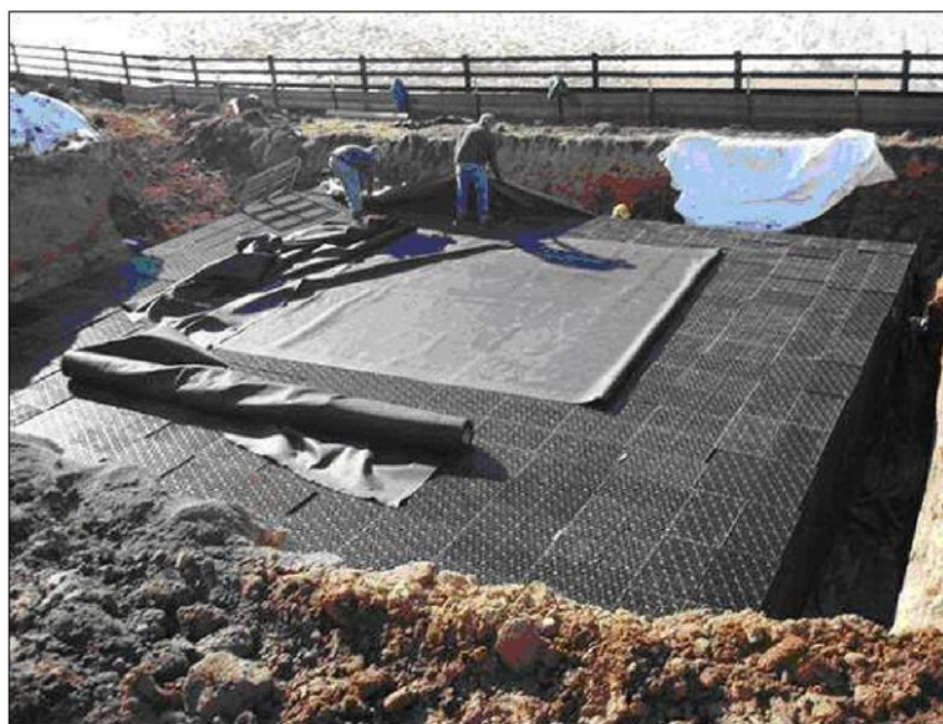
Figure 11.14. Example of Modular Units (Source: VADCR, 2011)
