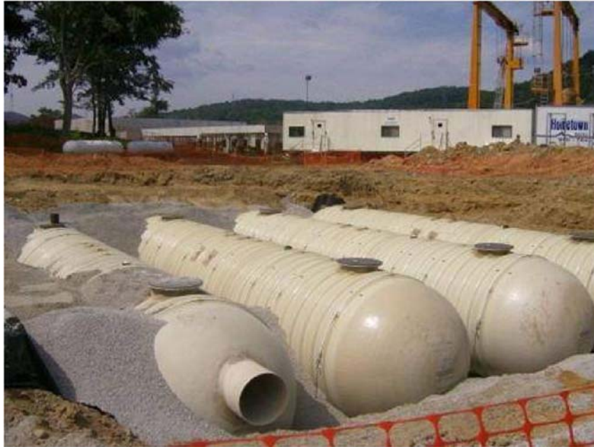
Figure 11.12. Example of Multiple Fiberglass Cisterns in Series (Source: VADCR, 2011)
