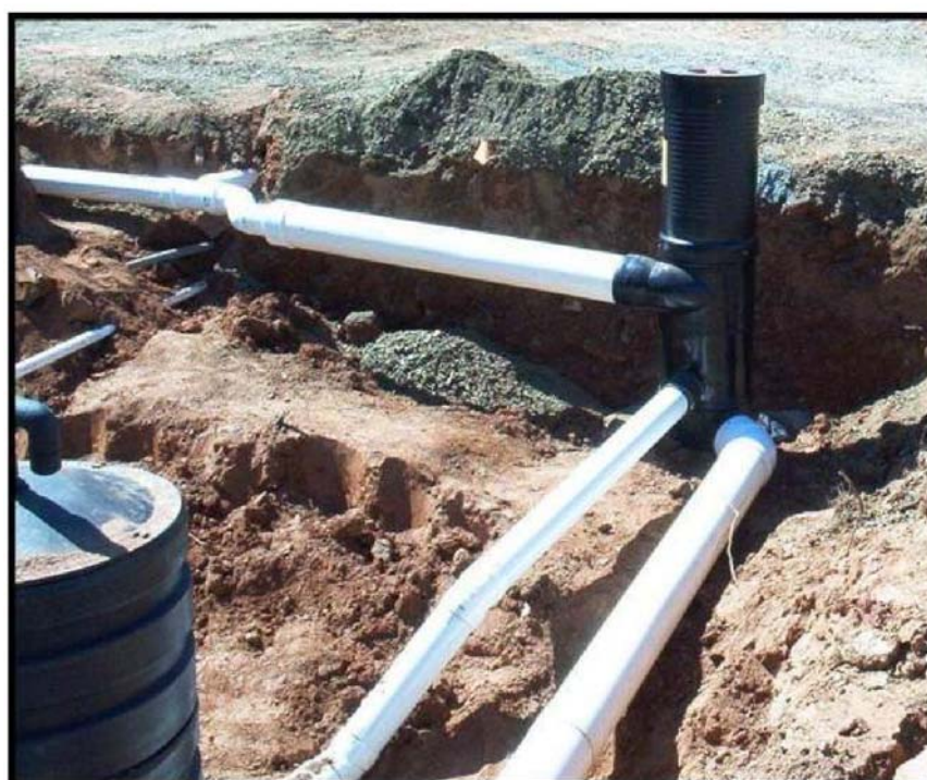
Figure 11.11. Installation of Vortex Filter prior to backfill (Source: VADCR, 2011)
