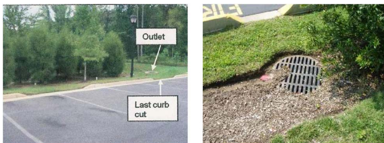
Figure 1.13. Examples of Short-Circuiting at Bioretention Facilities (source: VADCR, 2010)
